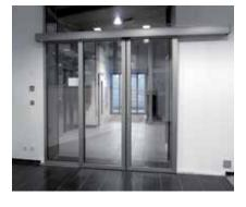
The combination of low "U" values, plus high resistance to currents of air, driving rain and wind, create a sliding door with optimum heat insulation.
